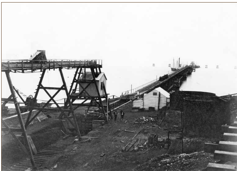
An early scene of the jetty at Hummock Hill about 1912. It shows a horse hauling a rake of loaded ore cars out onto the jetty for possible loading into the waiting ketch. J. Jobson.
