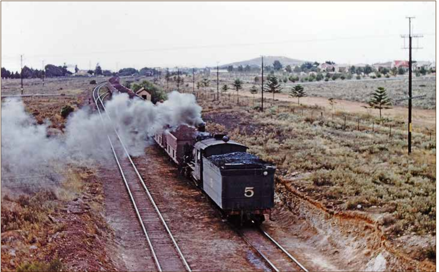
Small Baldwin No. 5 pushes a rake of loaded ore cars towards the unloading bins at Whyalla c.1956. BHP Archives.
