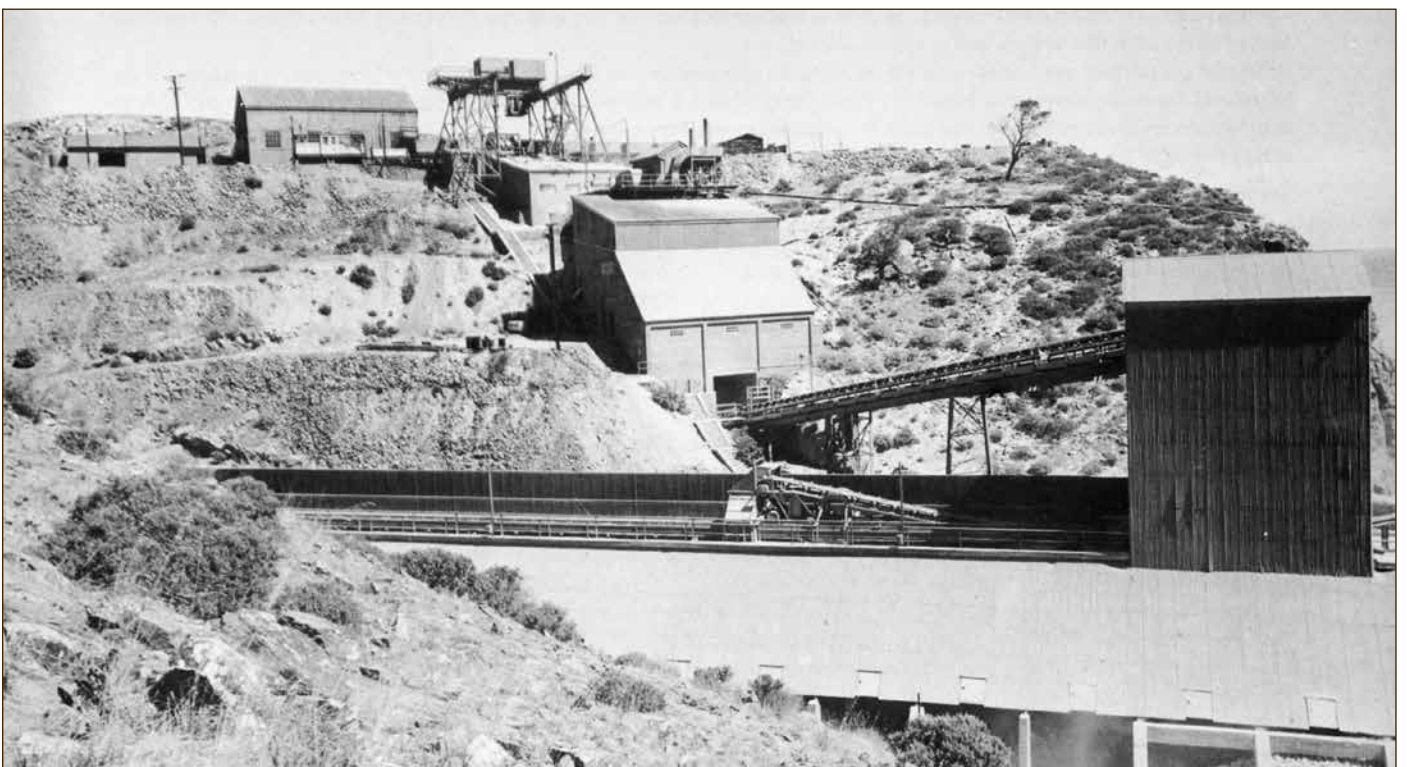
The Rapid Bay crusher and conveyor plant dwarfs an electric locomotive on the edge of the quarry. Taken during the 1950s this photograph clearly shows the extent of mining construction plant and equipment associated with BHP at Rapid Bay, just 50 miles south of Adelaide! BHP Archives.
