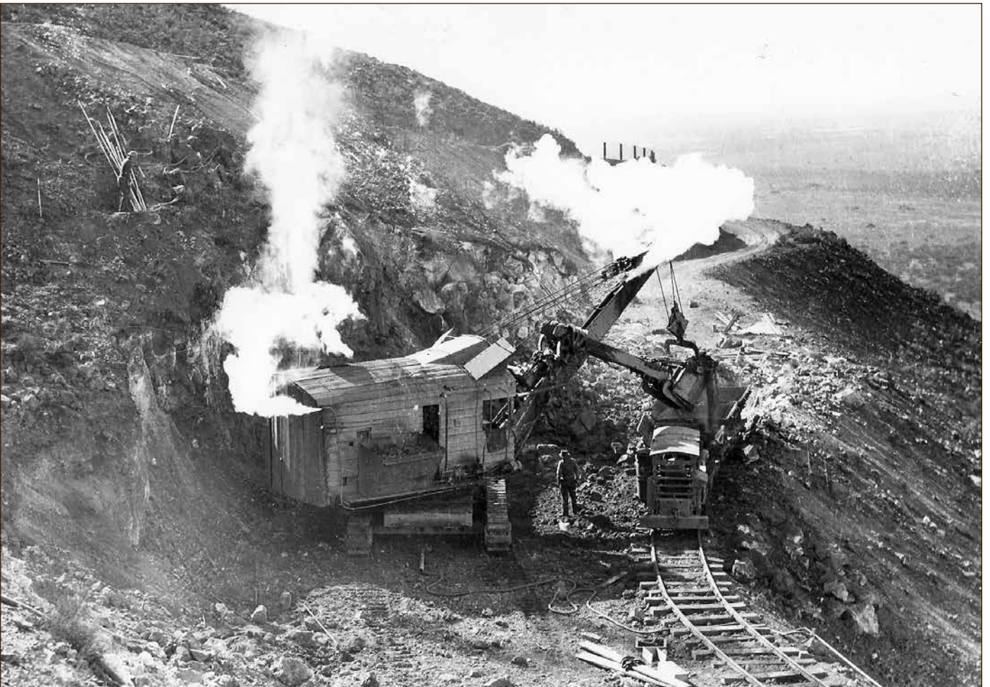
This 1928 scene shows another steam shovel loading a quarry train hauled by a Fordson kerosene locomotive. BHP Archives.
