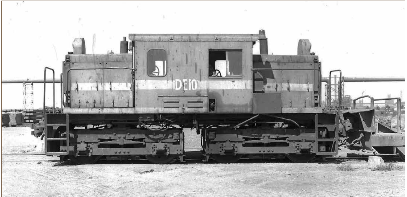
DE 10 in its final form. Once fitted with bogies off an electric locomotive, the general appearance of the original PE 1 was lost. It stands here in the moulding yard on 11/3/1975. BHP Archives.
