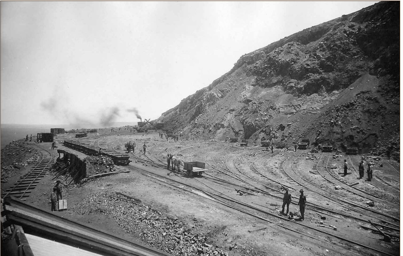
'A' quarry at Iron Monarch in 1920 shows steam shovels at work. Note the complex quarry trackwork. BHP Archives.
