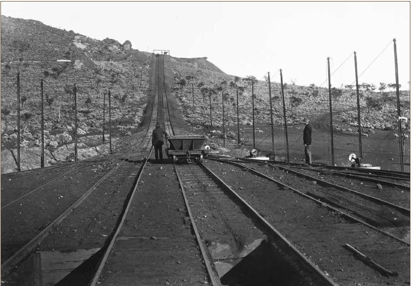
Empty trucks start their upgrade trip, from the unloading bins at Iron Monarch, to the quarry face during December 1914. J. Jobson.
