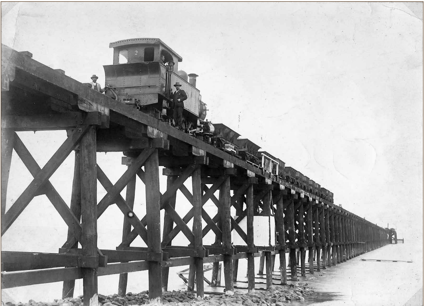
No. 2 shunts a string of cars onto the Hummock Hill jetty ore 1914. BHP Archives.
