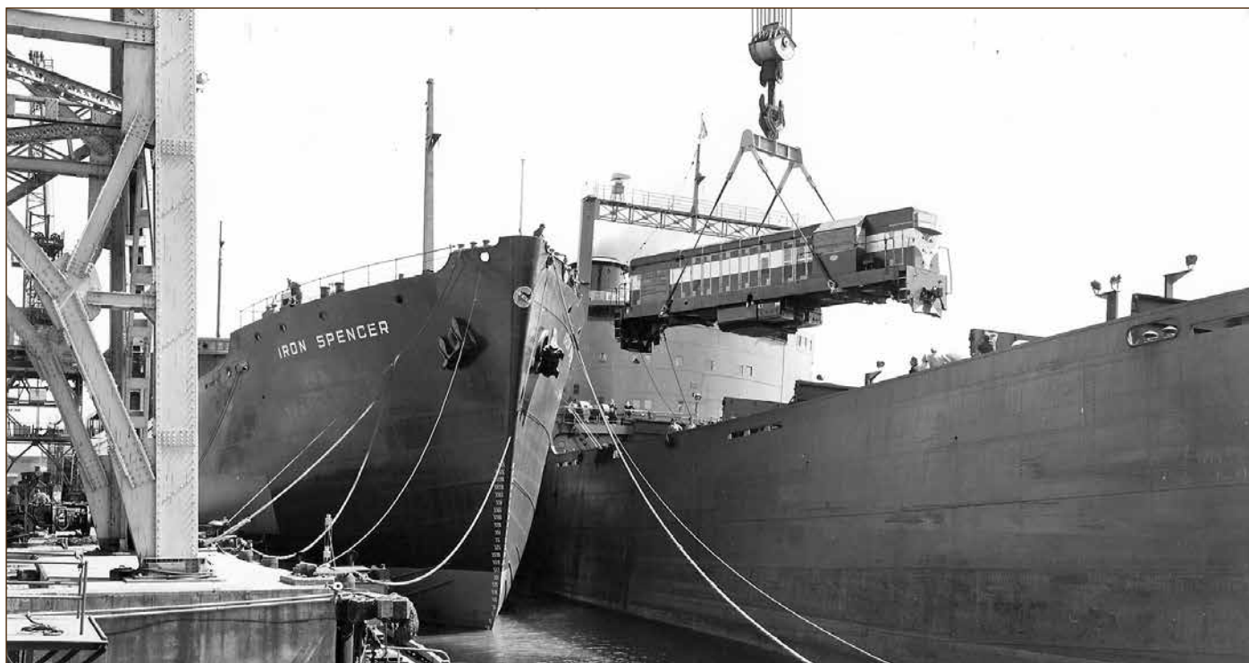
DE 01 is lifted by the 150 ton fitting-out wharf crane at Whyalla on 23 October 1956. DE 01 was deck cargo on SS 'Iron Whyalla', berthed next to SS 'Iron Spencer'. BHP Archives.
