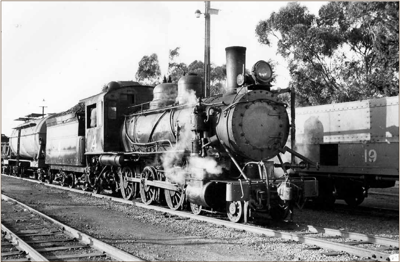
The last run of No. 4! A special steam hauled train operated over BHP's main lines to Iron Knob and Iron Baron over the weekend of 8-9 August 1964. (Above) No. 4 prepares to depart Whyalla working this special, while (below) it pauses for photographs enroute to Iron Knob. Both: D. Worth.
