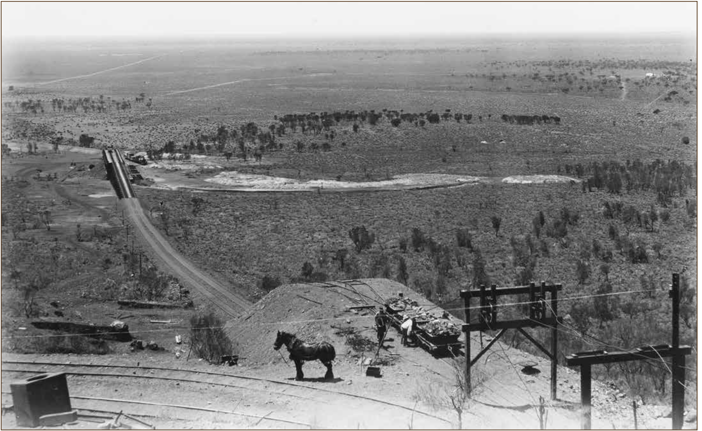
Three loaded four-wheeled incline trucks are prepared for the journey downhill to the bins at Iron Monarch during December 1914. J. Jobson.
