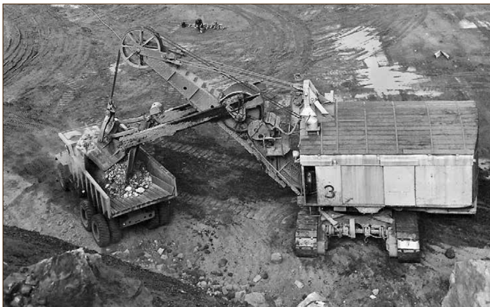
The unattractive result of the end of the quarry tramways. Electric shovel No. 3 loads a 'Mack' road truck in Iron Monarch, c.1960. BHP Archives.
